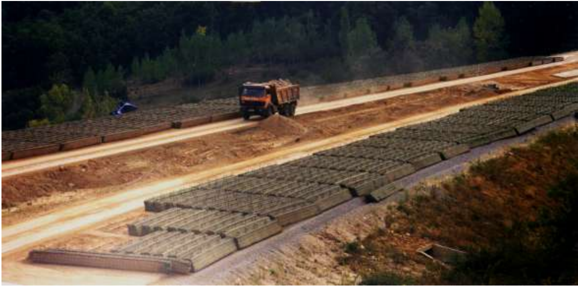
Geogreen Gabion wall in Ponferrada, Motorway Madrid-Coruña, Spain
