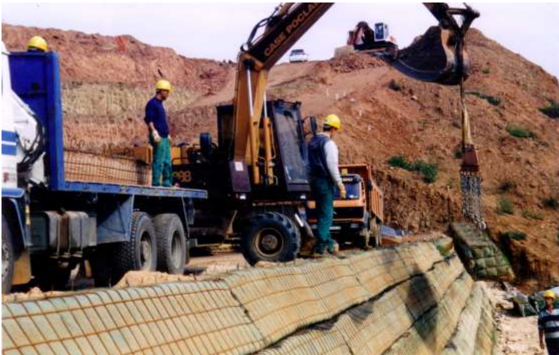
Geogreen Gabions being installed from Truck
