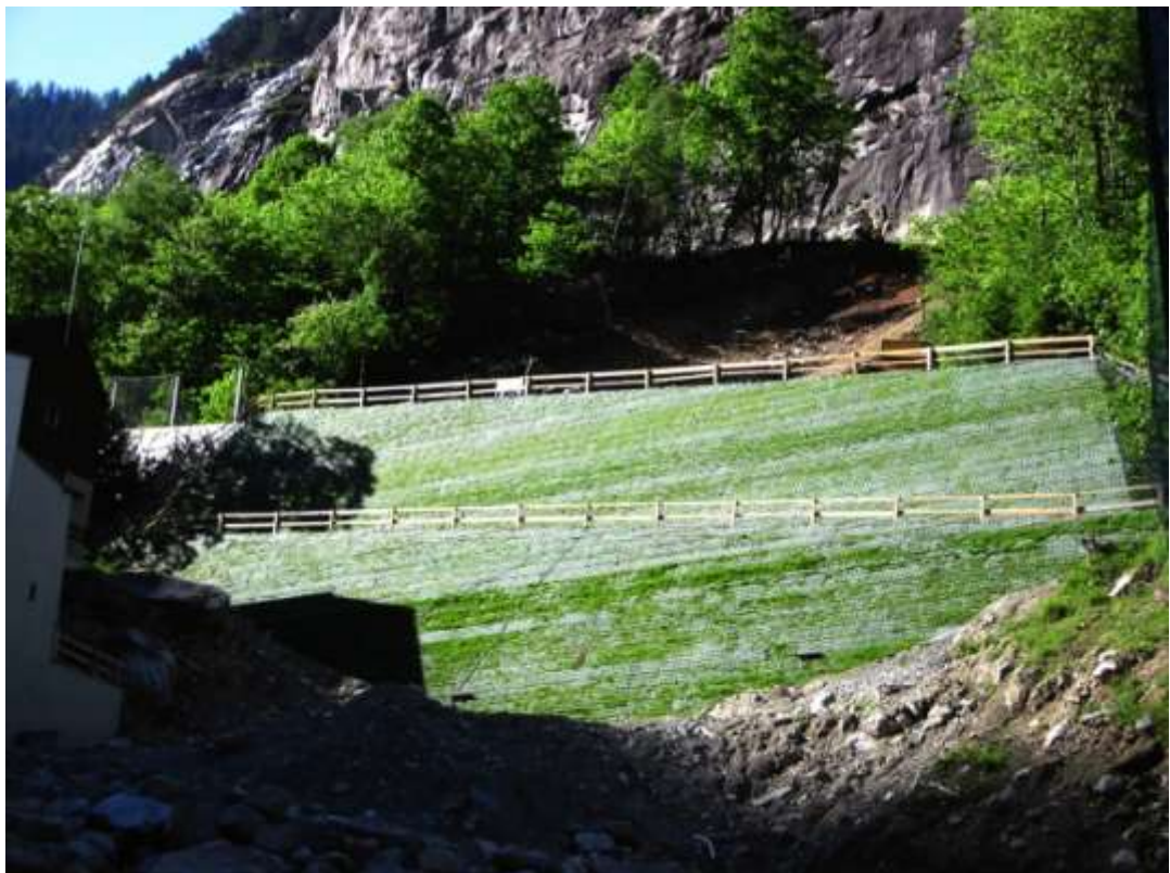
The 20 m high retaining wall is completed and getting hidden by grass plants.
