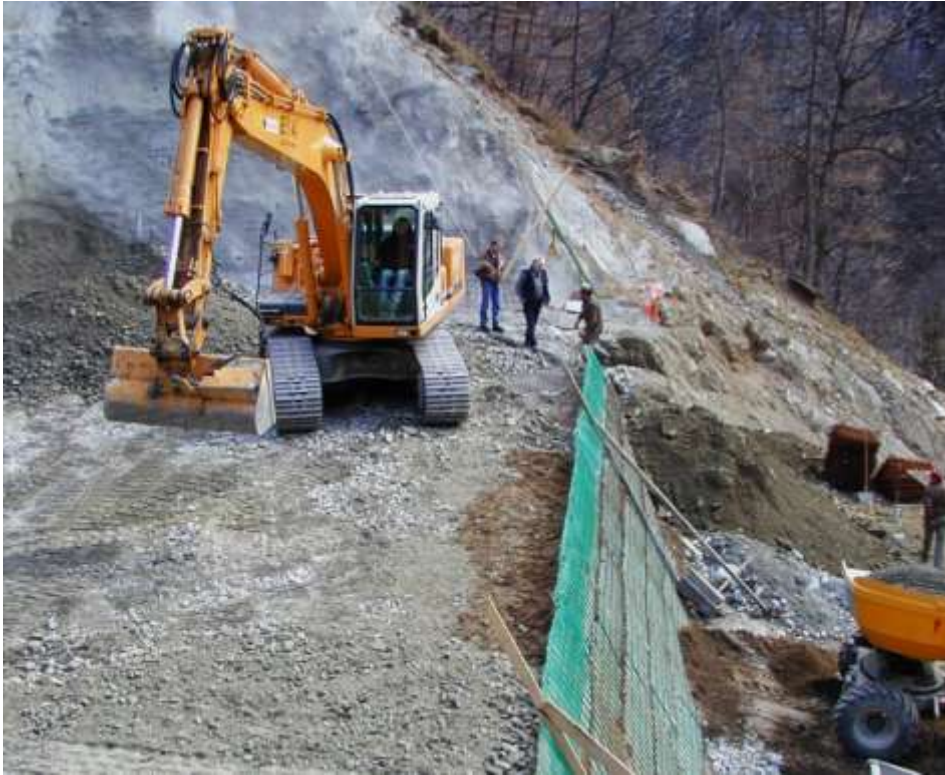
Geogreen Situ wall , under construction in Gondo, Switzerland.
