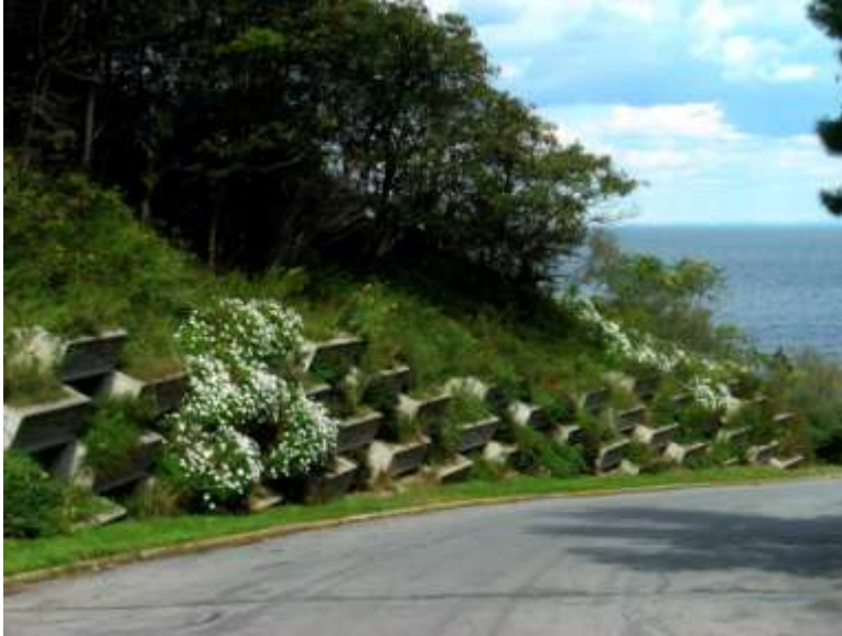
Evergreen GEO wall built in Port Jefferson, Long Island, New York
