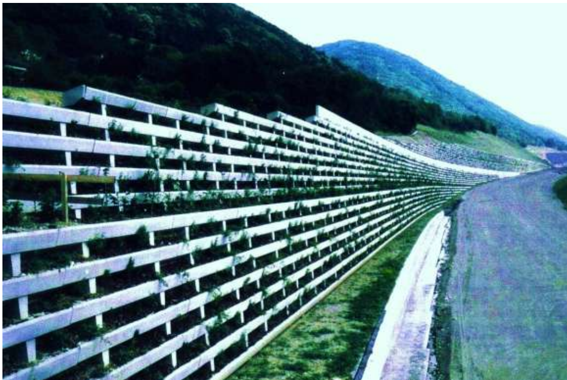
Motorway A 51, near Grenoble, France, high wall, about 6000m 2
