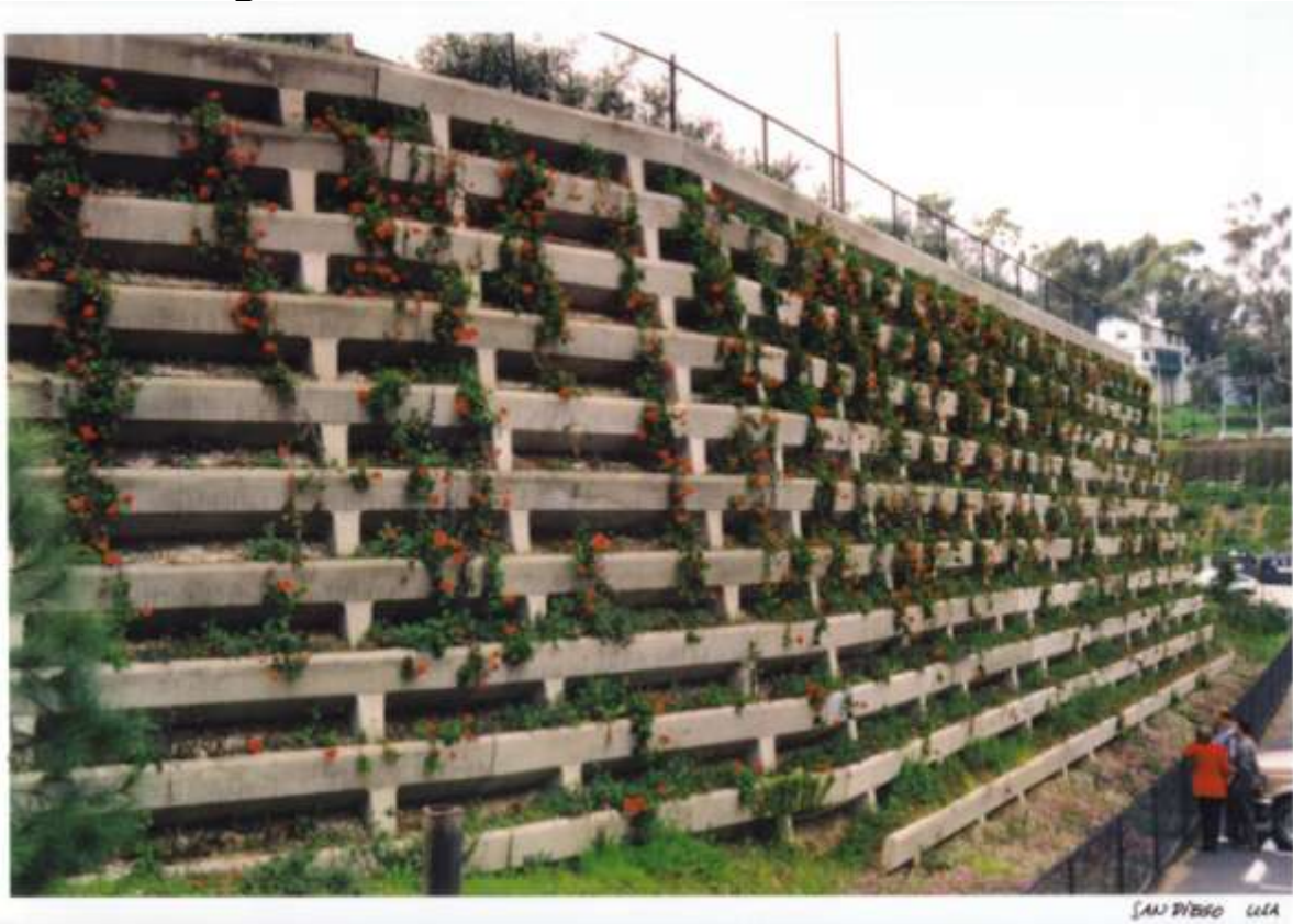
San Diego – Spring Street – for San Diego Metro Rail Parking, USA
