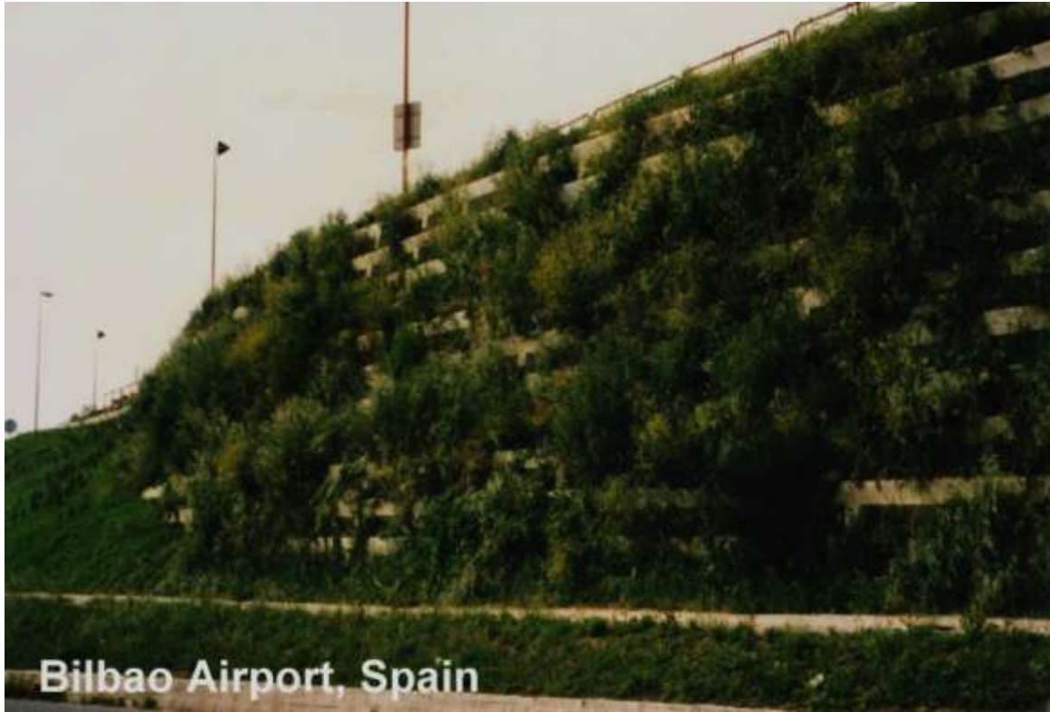
International Airport of Bilbao, Spain, Access Road, Wall about 10 m high
