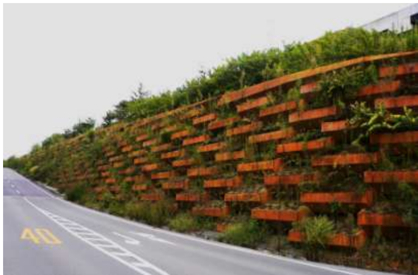
Evergreen Geo Wall built in Japan under a new Motorway
